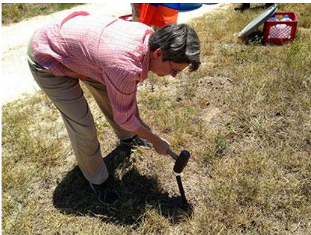
Sr. Kerstin Maria assisting with the installation of a water station in the desert near Falfurrias, Texas
